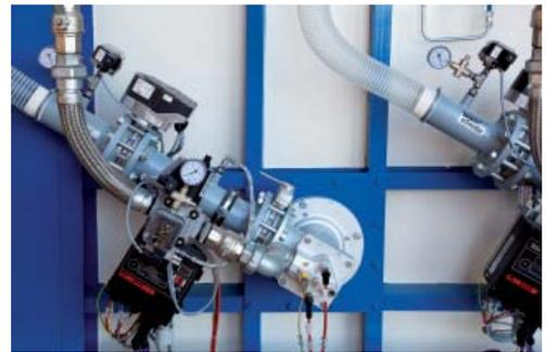
*20 gas-operated burners provide a total capacity of 9 megawatt*
