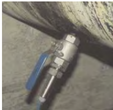
Flow measurement in discharge pipes Interruption-free assembling of the measurement device
